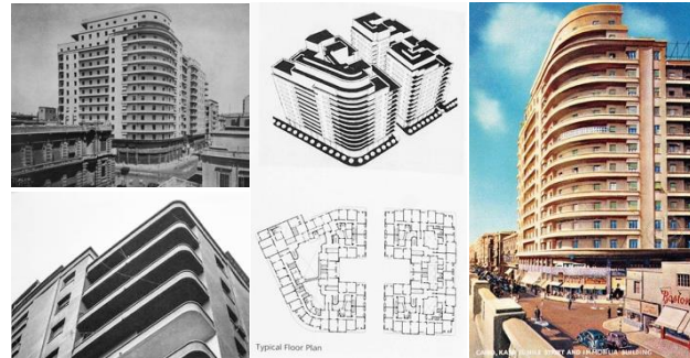
Figure (7): The Immobilya Building, Downtown Cairo, Max Edrie and Gaston Rossi, 1937-1940 Source: Harvard University. (n.d.); Noire, T. (n.d.).
