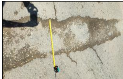
Fig. 14. Utility Patching No.1.
