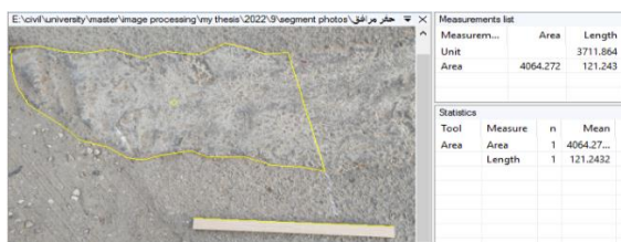
Fig. 42. Utility Patching No.1.
