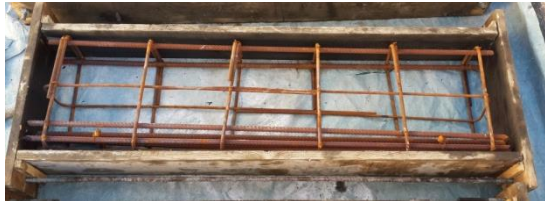
Fig. 4: Casting of deep beam
