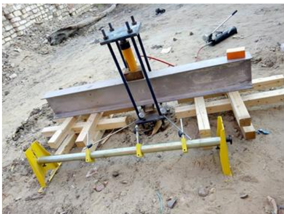
Figure (5): Field Helical Pile Test Setup.
