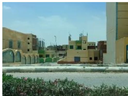
Figure 10: Unorganized Survey resulting building structure irregularity in heights.
