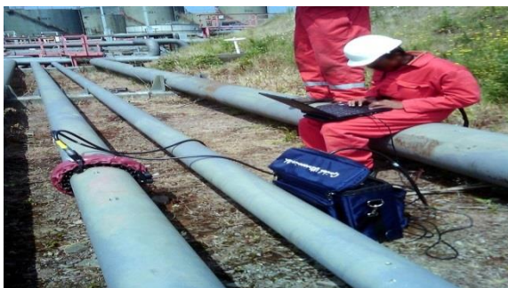
Figure 4: An example of pipeline inspection using guided wave testing (GWT).
