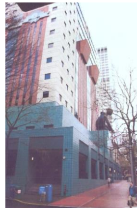
Fig. 4: Steps clad in bluish green ceramic tiles
