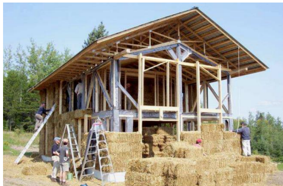
Fig. (6) Sustainable building: Straw bale [Edwin R.P. Keijsers, Sustainable building materials from rice straw]
