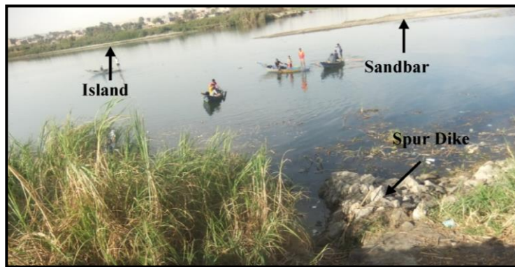
Figure 15: The Association of Local Deposition with Local Scour Sites in the Spur Dikes Area
