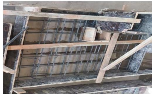
Fig. 1: Layout of slab with one opening
