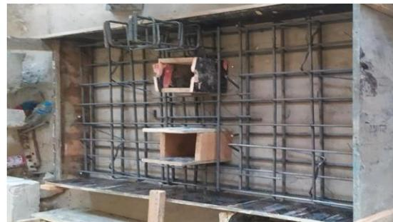
Fig. 2: Layout of slab with two openings
