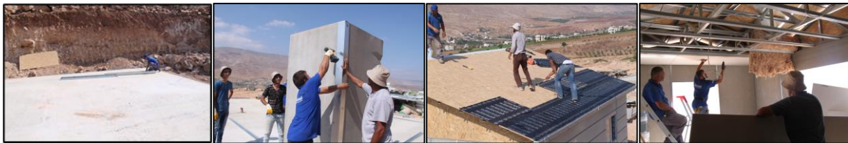
Figure 4. Steps to implement prefab houses source Diyarna Company
