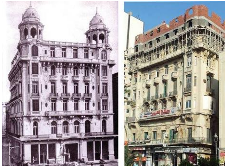
Fig (4) Violations of heritage buildings within adding some floors
