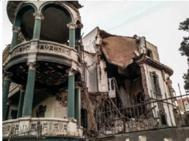
Fig (3) Demolition of heritage buildings during the January 2011 revolution
