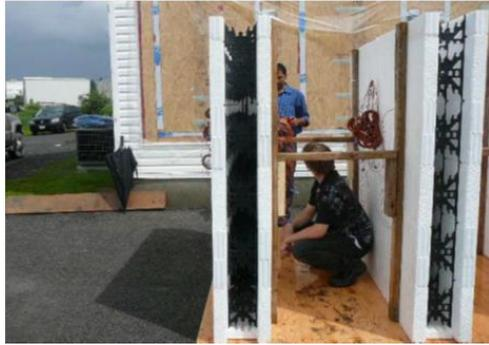
Fig. 7. Insulated Concrete Formwork (ICF) [12]
