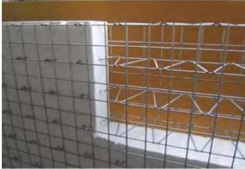
Fig. 8. EPS core panel detail [13]
