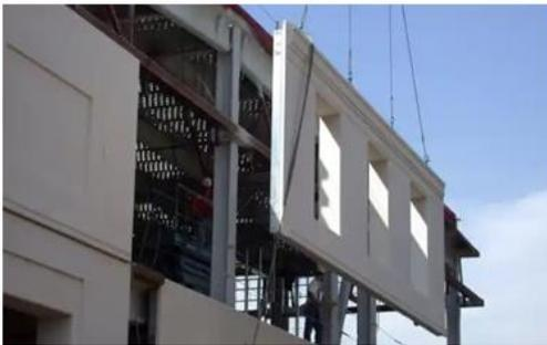
Fig. 3. Prefabricated linear walls [17]
