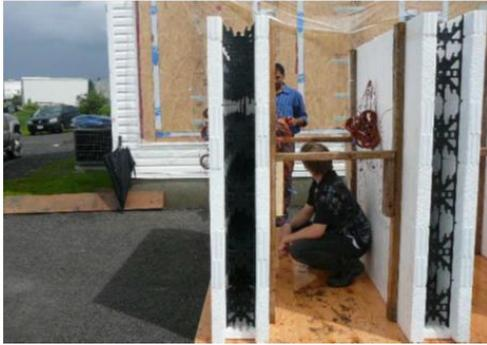
Fig. 7. Insulated Concrete Formwork (ICF) [12]
