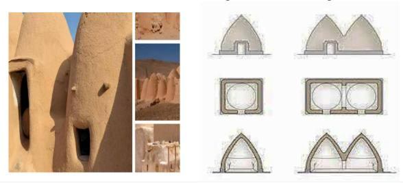
Fig 3 Show the important typologies of corbelled domes which has been distinguished: by the old hypogean developments
