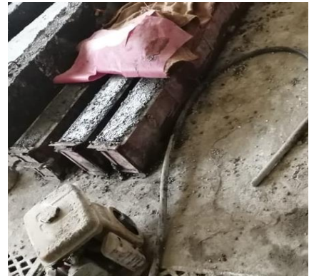
Fig. 6. Stage 4: Four lightweight concrete beams
