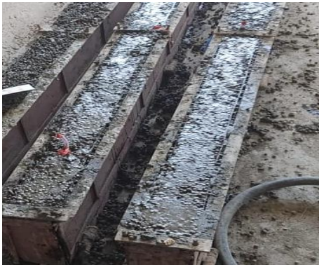
Fig. 5. Stage 3: Two lightweight concrete beams
