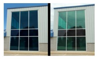
Fig.8 The effect of lighting on the color and transparency of glass used with photochromic technology. <u>https://www.bdcnetwork.com/ppg-pleotint-co-marketenvironmentally-adaptive-glazing-technology-low-eglass</u>
