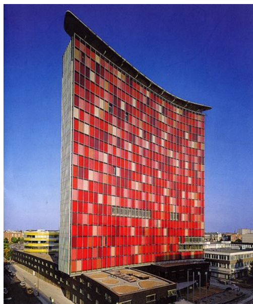
Figure2: GSW building, Intelligent façade , Active façade, Ability to learn and respond in time Combines automatic and occupant control(10)
