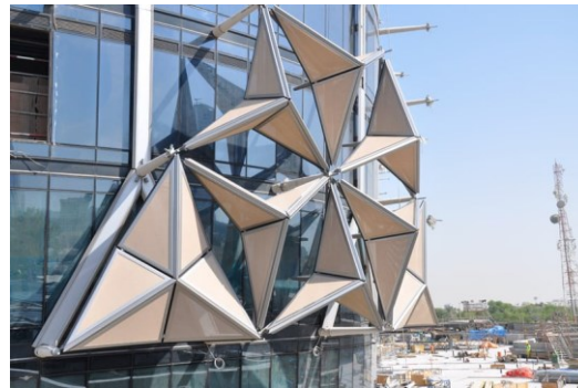
Figure3: Al-bahar tower- Kinetic façade- Working with mechanical systems Acting based on outdoor environment condition- Moveable façade
