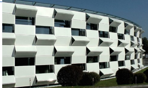
Figure 7: Kiefer Technic showroom -Responsive façade- Thermochromic polymers- smart windows- Similar performance characteristics to an ‘intelligent’ façade Usage of sensors, actuators, and control devices
