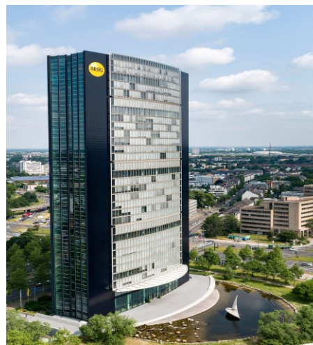
Figure 8: The administrative building in Germany (ARAG VERSICHERUNG), the use of the front of the box air column to make differences in pressure and benefit from natural ventilation in tall buildings, and by dividing the facade, it works as ventilation columns linked to openings every eight floors.
