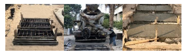
Fig. 3. Pouring concrete for beam specimen
