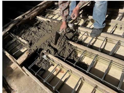
Figure 5- Casting the fresh concrete.
