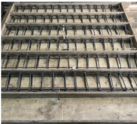
Figure 4- Wooden forms for specimens.
