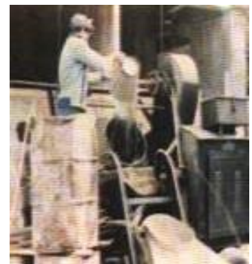
Figure (8): Wrong gravel calibration method using the loader Figure (9): Wrong water calibration method using a bucket (Source: ref. [7]).
