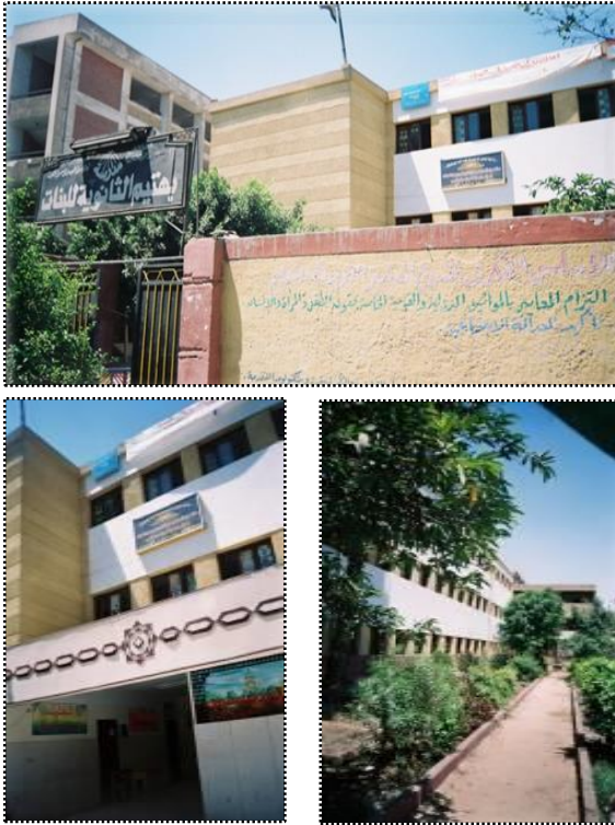
Figure (14) a,b: The front facade of Bahtem Secondary School for Girls (Source: Author).
