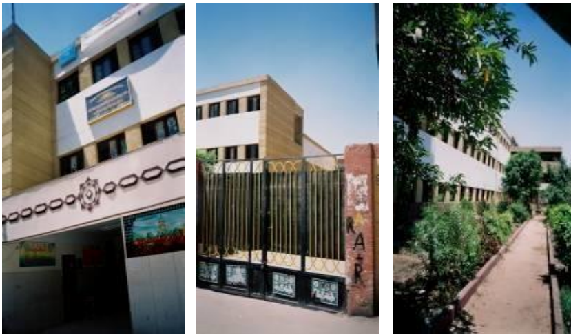
Figure (26): External perspective of the school after the process of maintenance, development and rehabilitation (Source: Author).
