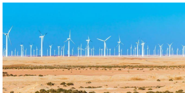
Figure 6. Wind Farm, Zafarana- Egypt
