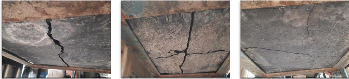
Figure 9. The failure mechanism of different concrete slabs (NC, MMGS, and MMGSM).
