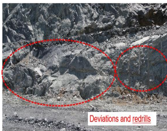
Figure 12 Borehole deviation and redrills
