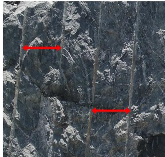
Figure 13 Improved presplit drilling and blasting
