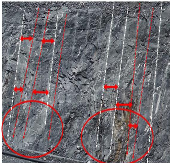
Figure 11 Common presplit drilling errors.
