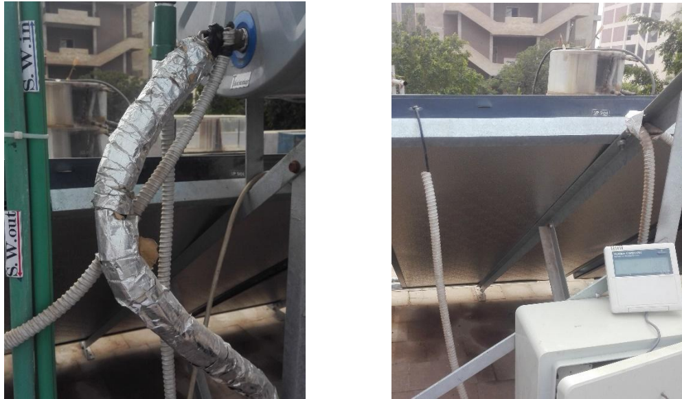
Fig.(1) Thermocouples Connections.
