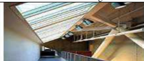
Figure 3 shows glass panels that provide natural lighting
