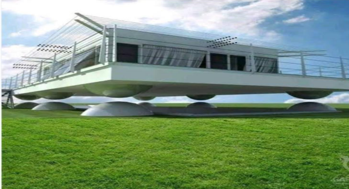
Figure 7: Levitating house by deploying airbags. ( http://award.designtoimprovelife.dk/nomination/243 )
