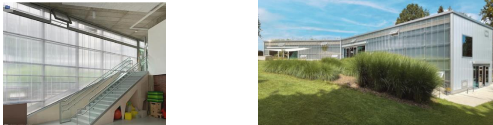
Fig (6) polycarbonate panels used in the holly facades of daycare center project, Karoline Goldhofer, in Memmingen, Germany. [60]
