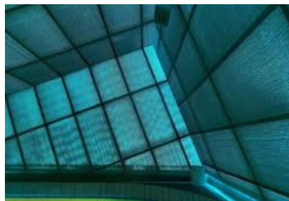
Fig (7) transmitting concrete salt crystals LUCEM in the public swimming pool “Obermaintherme” in the Bavarian city in Germany, 2016
