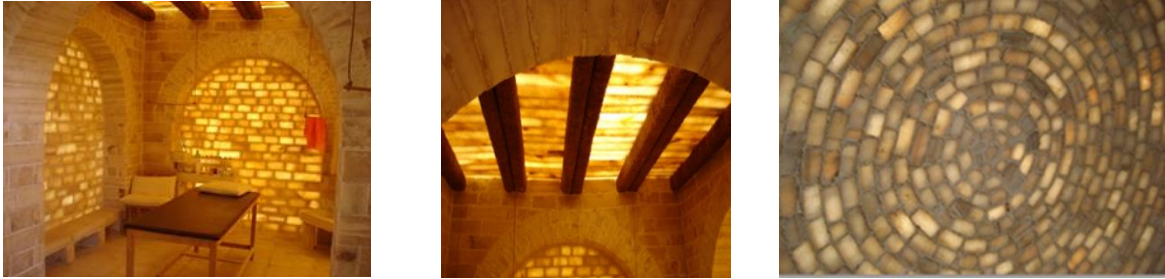
Fig (3) using transparent salt bricks on the outer envelope of the building in Siwa Source: Researcher
