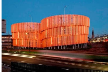
Fig (12) Parking Garage building in Zutphen made out of Translucent Wood_©foreco.nl
