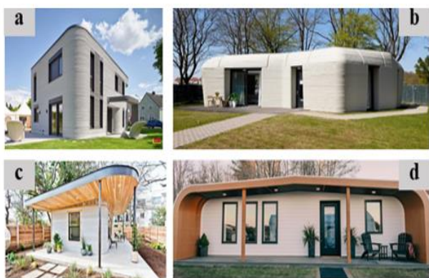
Fig 17 (a) Mense-korte’s Germany 3D printed house [27]. (b) Milestone 3d printed house [28], (c) Chicon house, ICON’s 3D Printed House in Texas [29]. (d) The first bio-based 3D-printed home in the world, biohome3D [30].
