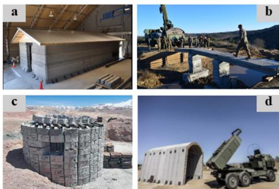
Fig 20. (a) 3D Printed Barracks hut [36], (b) the 3D printed pedestrian bridge [37], (c) 3D printed bunker [37], (d) vehicle 3d printed hide truck [37].
