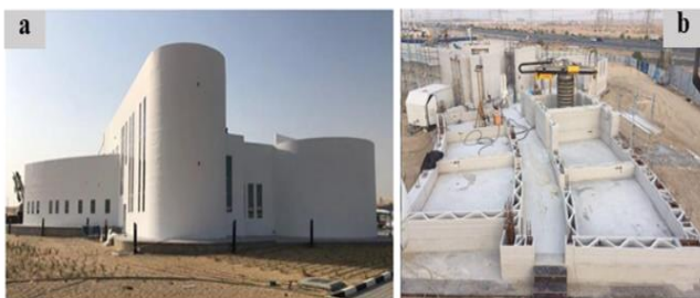
Fig 14. world's largest 3d printed office in Dubai [21].
