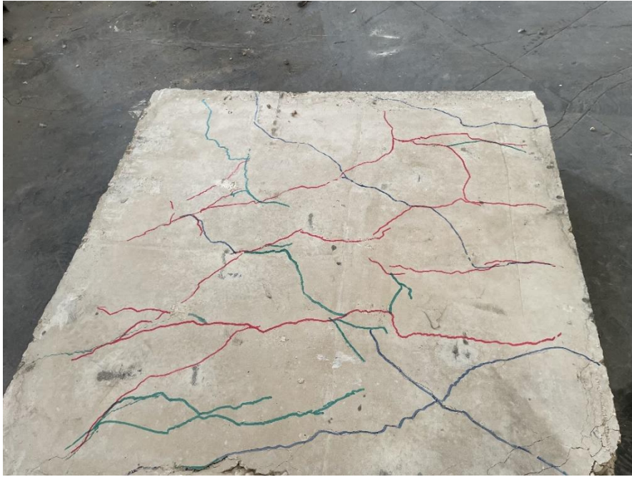
Fig. 9. Crack pattern of slab (S1) (Reference slab).
