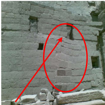
Fig. (8) Differential tendency on the walls of Luxor temple
