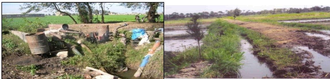
Fig. 3: individual privet pumps and the earthen Mesqa in traditional surface irrigation
