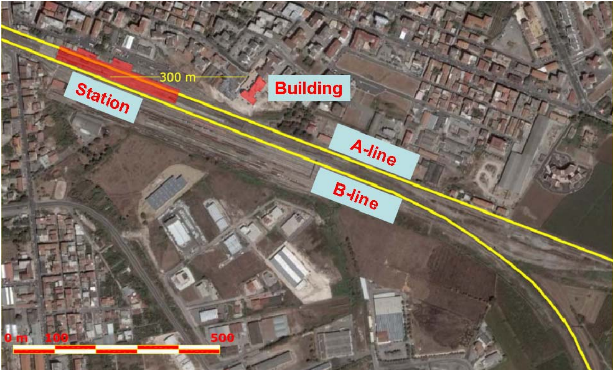
Fig.1. Aerial photogrammetry of area under investigation. [5]
