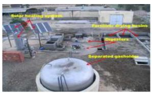
Fig. (\*\*): biogas and bio-fertilizer production system
