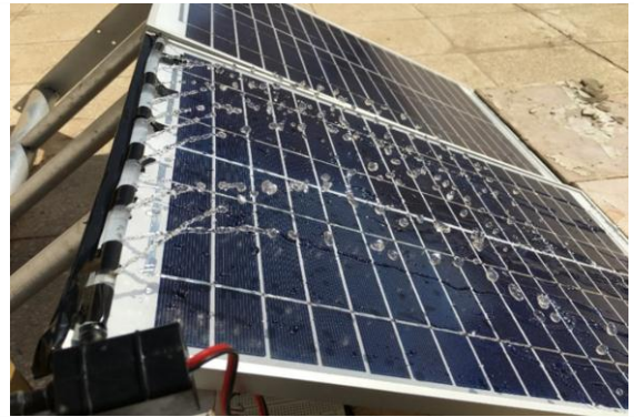
Figure 4:experiment 1. Water spray cooling technique using power pump connected to pipe line with holes at the panel's front side.
