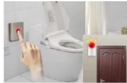
Figure 17: Bathroom emergency bell Source: www.nationalcallsystems.com
