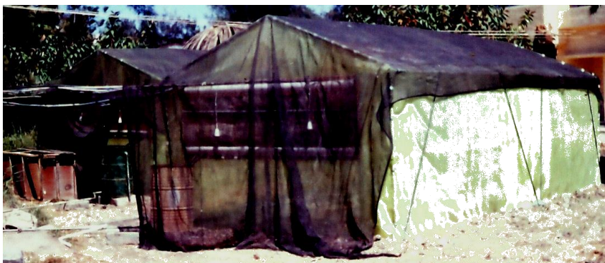
Fig (2). The two greenhouses covered with blanket net 60% to reduce the solar radiation incident.
