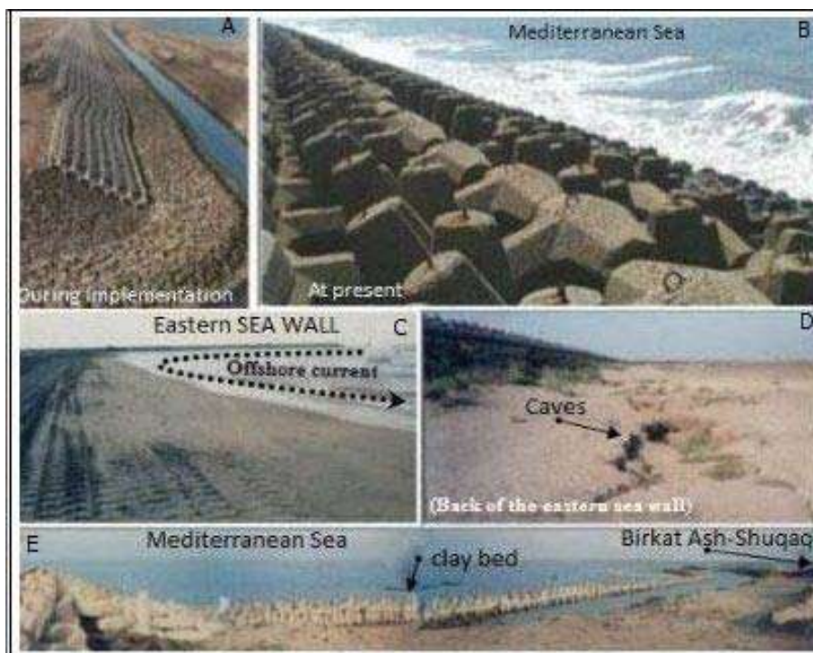
Figure. 2: Erosion process around the eastern sea wall of Rosetta promontory.
