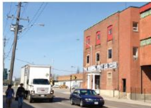
8 The original Rumpel Felt Building has cultural heritage value and is intended to be adaptively reused as part of the Transit Hub plan.
