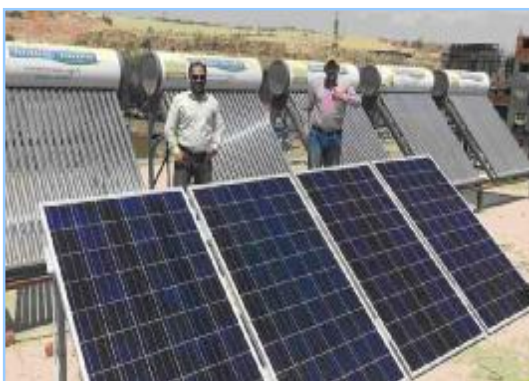
Figure 23, Installing Solar panels
