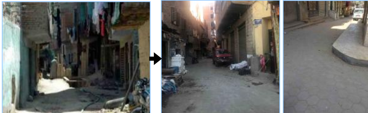
Figure 16, Ezzbet el Nasr before and after paving of street and installing proper infrastructure
