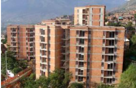
Figure 4, Juan Bobo re-housing project
