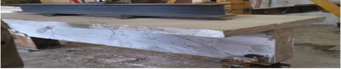
Beam (e) flange width equal 750 mm-splitting failure
