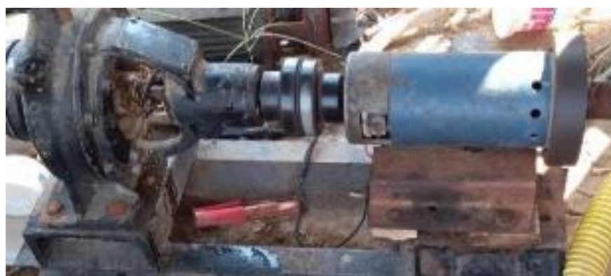
Fig. 4. Connection between the centrifugal pump and the DC motor
