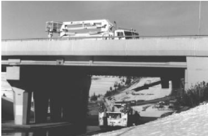
FIGURE 7. THE BEDDINGTON BRIDGE, CANADA.
