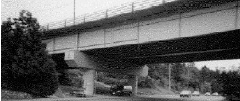
FIGURE 8. PORTAGE CREEK BRIDGE.
