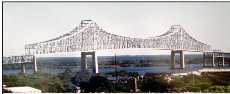
FIGURE 3. COMMODORE BARRY BRIDGE THROUGH-TRUSS STRUCTURE.
