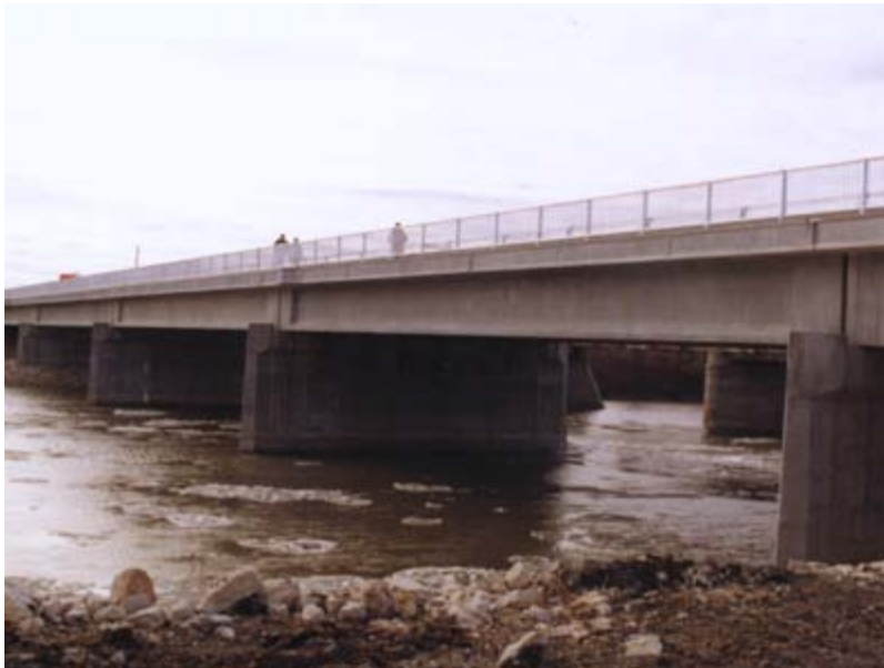
FIGURE 12. OVERVIEW OF TAYLOR'S BRIDGE [23].
