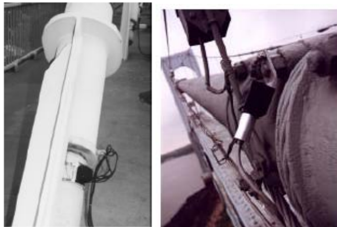
FIGURE 2. MOUNTING ACOUSTIC EMISSION SENSORS ON POST-TENSIONED TENDONS.
