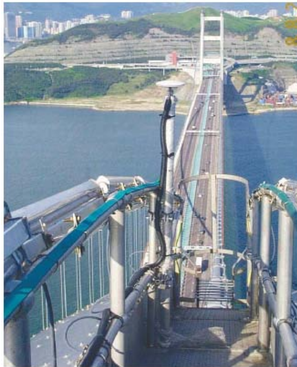
FIGURE 17. TOWER TOP RECEIVER ON TSING MA BRIDGE.
