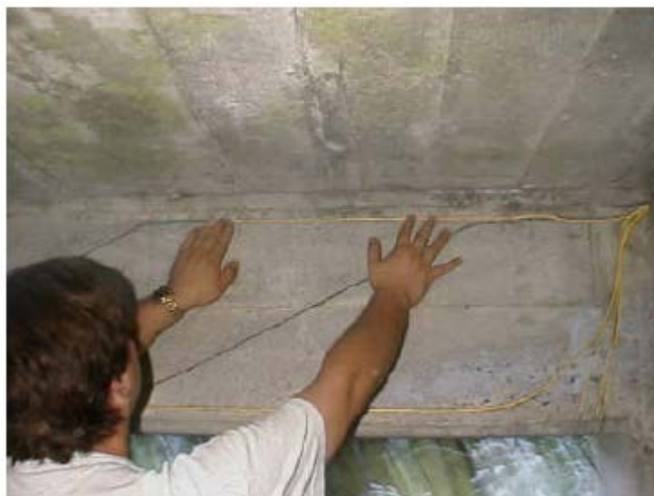
FIGURE 15. INSTALLATION OF LONG GAUGE LENGTH SENSOR INTO THE BEAMS.
