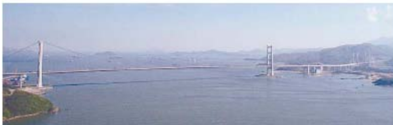
FIGURE 16. TSING MA BRIDGE.
