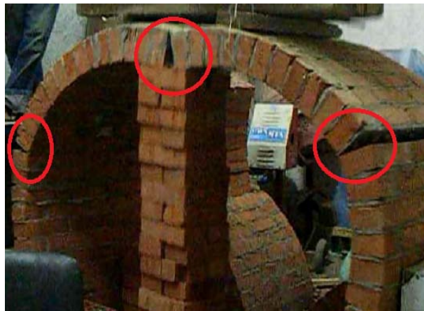
Figure 9 Control masonry vaults failure pattern.
