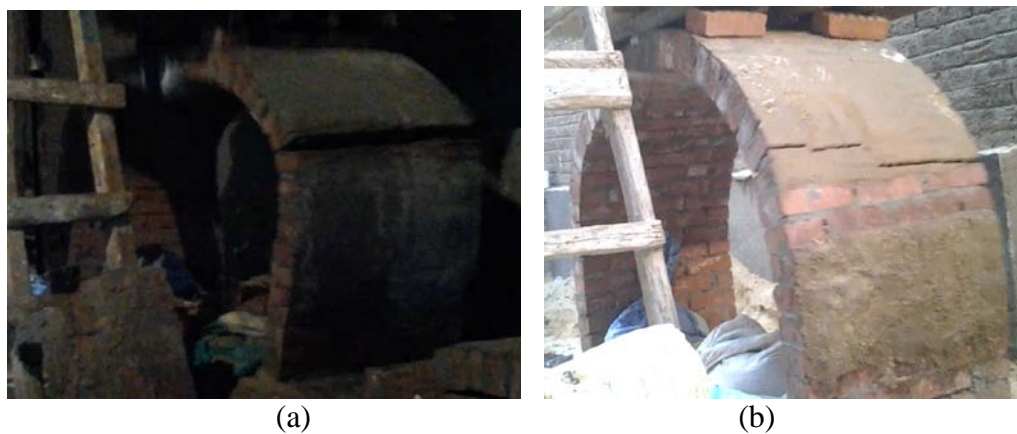
Figure 14 Mode of failure for vaults strengthened by (a) ferro-cement wire mesh, (b) polyester mortar
