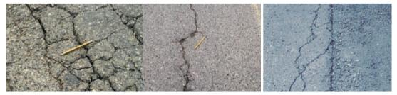
Figures (2): shows the different types of cracks; alligator (fatigue) cracking, longitudinal cracks and non-wheel path cracks.
