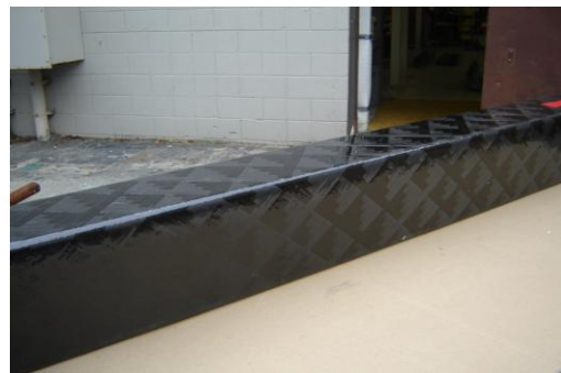
Figure (2d): Completed Beam after Filament Winding .
