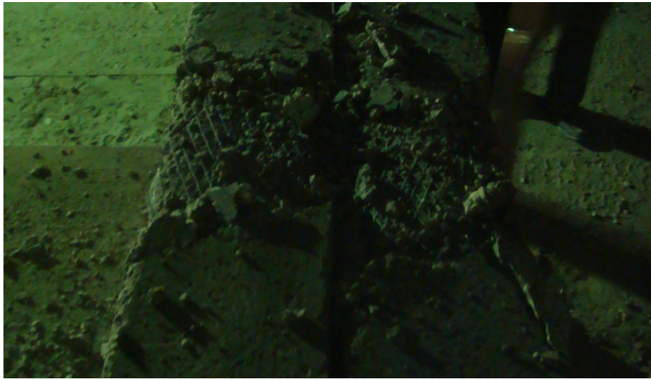
Figure 11-A: Details of Concrete model penetration.
