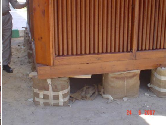
Fig. (19) Wall panels on foundation
