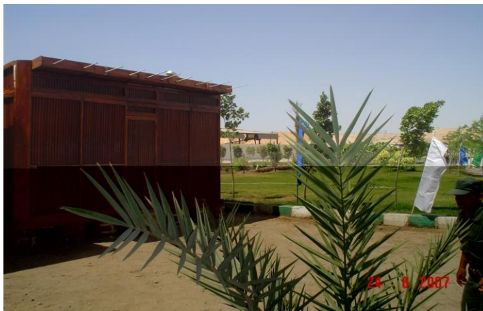
Fig (12) general view shows the tension cables
