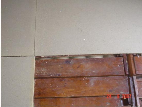
Fig. (18) Floor decking
