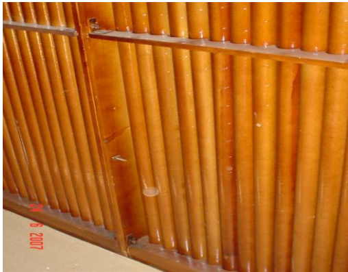
Fig. (14) Wall panels and bracing
