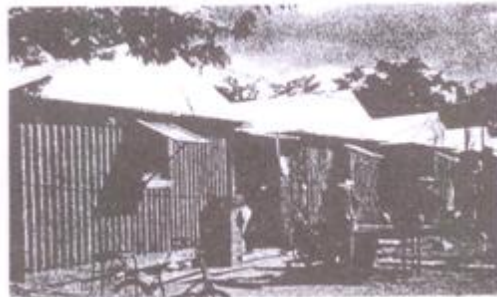
Figure (3) Exterior view for the shelter
