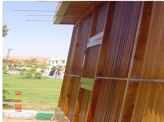
Fig. (15) Wall panels and roof panels
