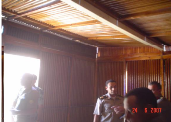
Fig (7) Indoor view shows the roof panels with wall panels
