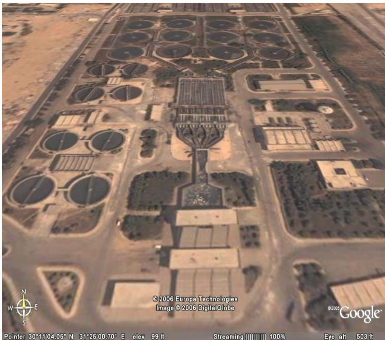
Photo (1) General layout of the treatment plant f the Al-Berka.
