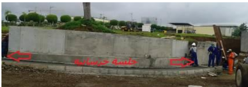
Fig. 6 the concrete mural involved in the research.
